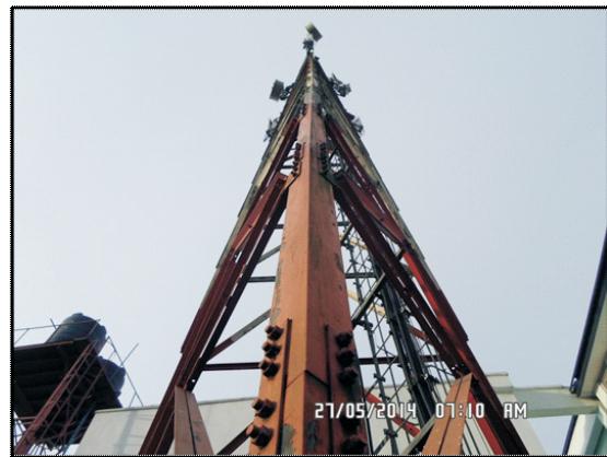
TOWER MAINTENANCE ACTIVITIES IN AN AIRTEL MANAGED SITE
