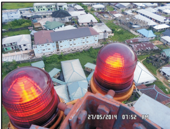
TOWER MAINTENANCE SERVICES – AVIATION WARNING LIGHT
